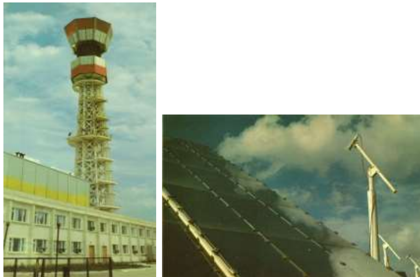
Fig.10. The tower of height 89 m and optical probe for controlling the turn of heliostats in two planes are shown in photos; a number of heliostats is 1600, size 5 \times 5 \text{ m}^2
